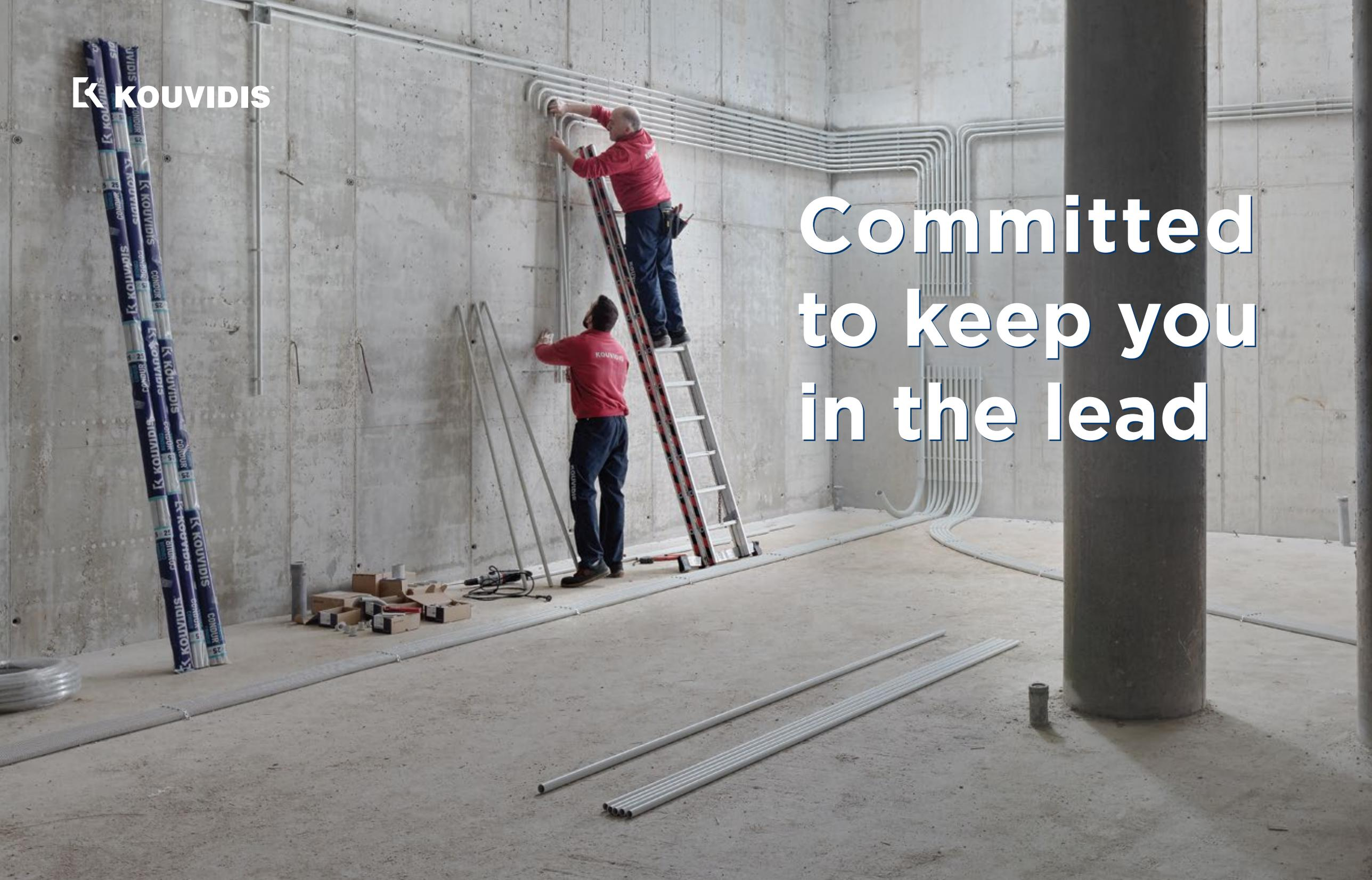
A photograph of two construction workers in red shirts and blue pants installing white conduits in a concrete room. One worker is on a ladder, and the other is on the ground. Bundles of conduits are stacked on the left, and several long conduits lie on the floor in the foreground. The room has concrete walls and a large pillar on the right.
